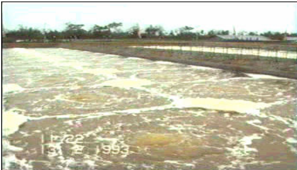
FIG 2 : JetHelix® in operation : Waste water treatment plant, Indonesia
